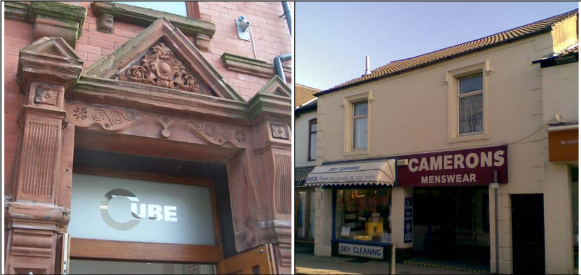
FIGURE 77. INTERESTING ARCHITECTURAL DETAILS
