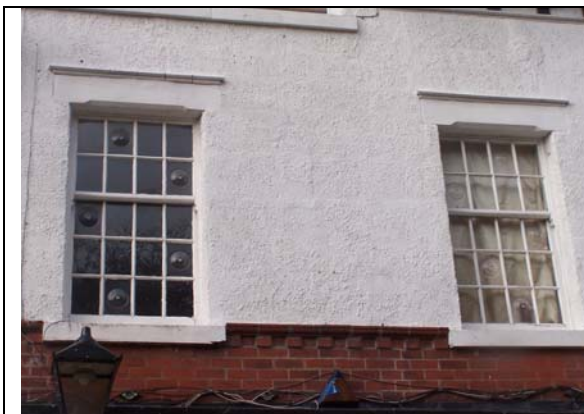
FIGURE 69. GOOD EXAMPLE OF SASH AND CASEMENT WINDOWS
