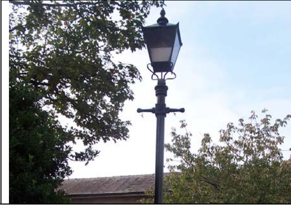
FIGURE 41. TRADITIONAL SMALL SCALE LANTERN STYLE STREET LIGHTING
