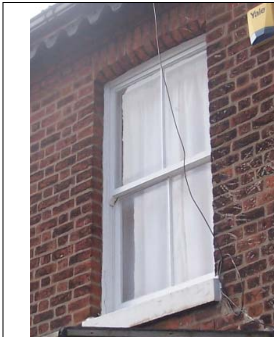
FIGURE 91. EXAMPLE OF REPLACEMENT TIMBER SASH AND CASEMENT WINDOW
