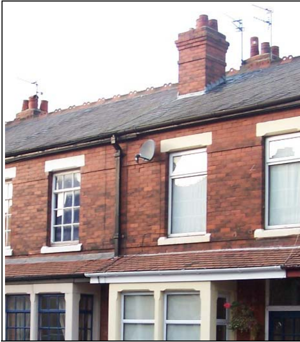
FIGURE 95. ORIGINAL WELSH SLATES
