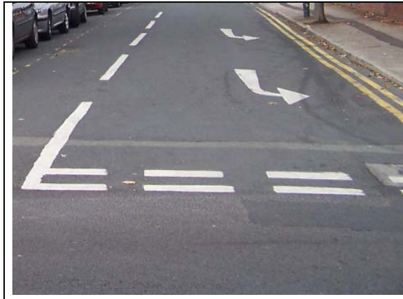
FIGURE 44. TARMAC ROAD AND CONCRETE SLAB PAVEMENT
