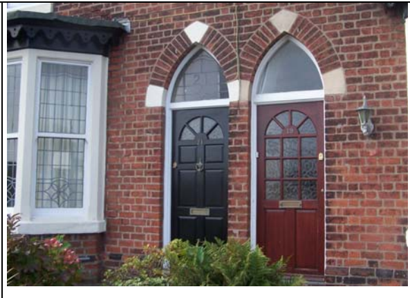
FIGURE 68. EXAMPLE OF SLIGHTLY RECESSED DOORWAYS
