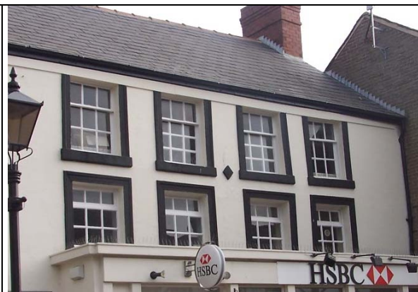
FIGURE 70. GOOD EXAMPLE OF SASH AND CASEMENT WINDOWS
