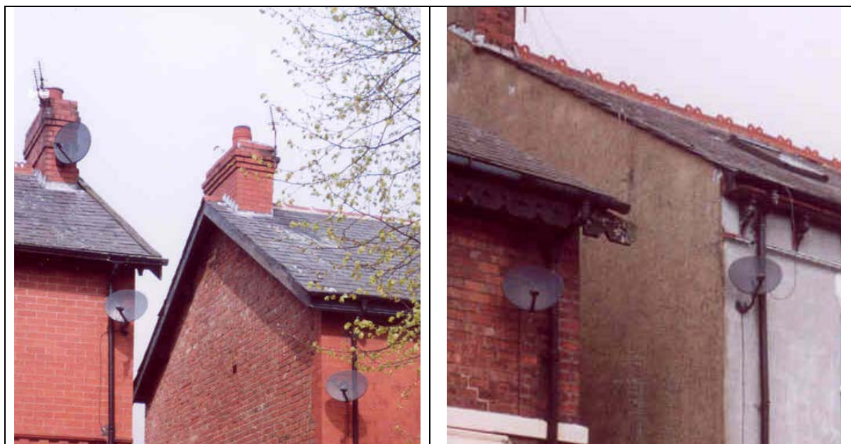
FIGURE 93. EXAMPLE OF SATELLITE DISH ON FRONT ELEVATION
