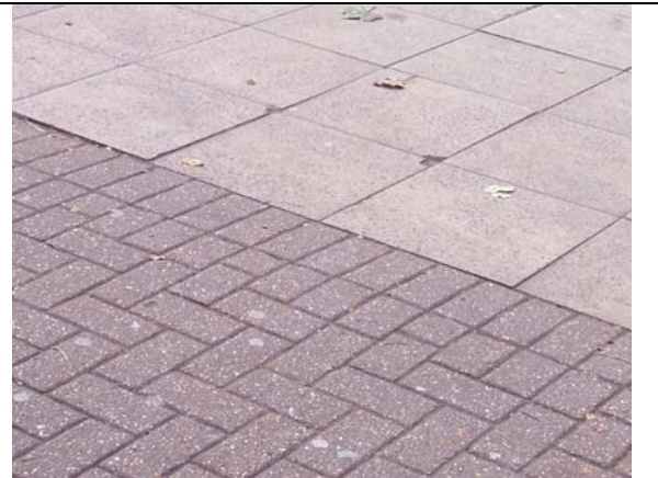
FIGURE 45. MODERN SETT STYLE PAVEMENT SURFACE, ALONG WITH LARGER MODERN PAVING SLAB
