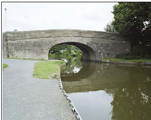
FIGURE 39. CANAL BRIDGE (NO. 62)
