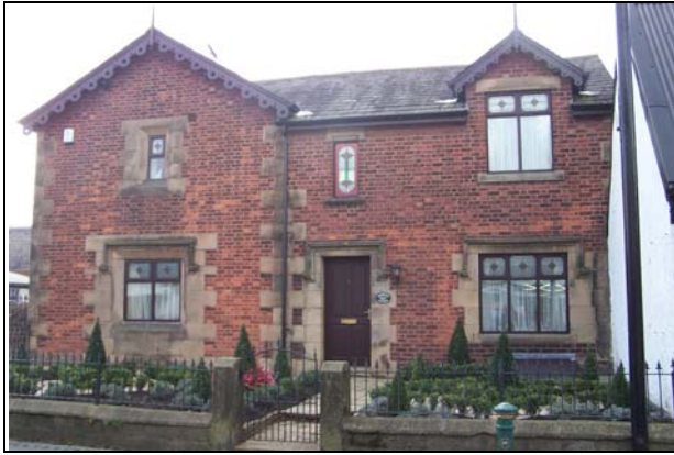
FIGURE 93. RESIDENTIAL PROPERTY ON HIGH STREET
