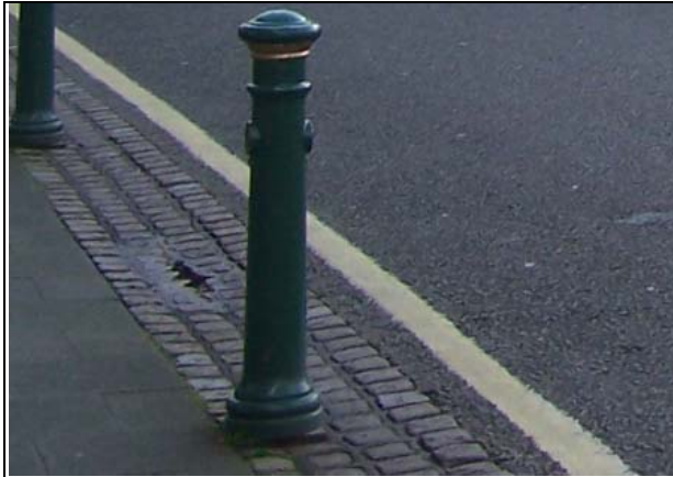
FIGURE 72. A CONCRETE PAVEMENT, SETS FOR THE GUTTER, AND A TARMAC ROAD, HIGH STREET
