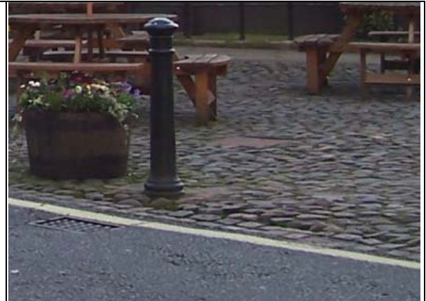
FIGURE 73. COBBLES IN THE MARKET PLACE, OUTSIDE ROYAL OAK HOTEL, HIGH STREET
