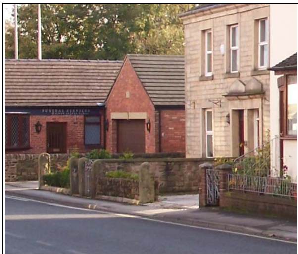
FIGURE 116. FRONT GARDEN LOST IN FAVOUR OF OFF STREET PARKING, LIABLE TO INCREASE FLOODING
