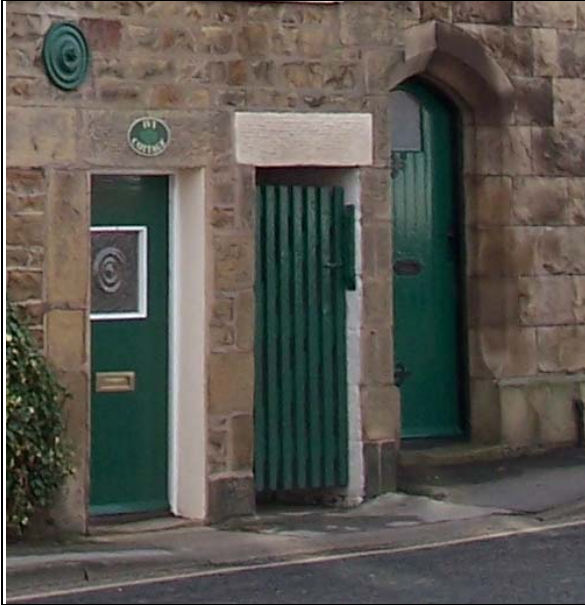
FIGURE 104. TIMBER DOORS, BRIDGE STREET
