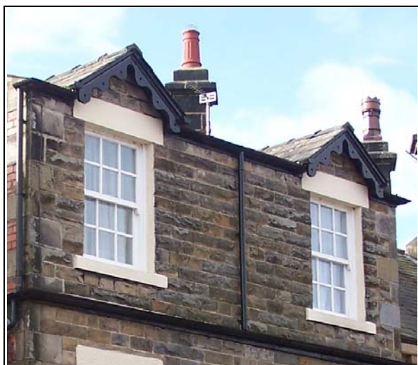
FIGURE 102. SASH AND CASEMENT WINDOWS, BRIDGE STREET
