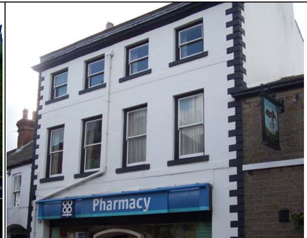
FIGURE 92. RESIDENTIAL UPPER FLOORS OF COMMERCIAL PROPERTY, HIGH STREET
