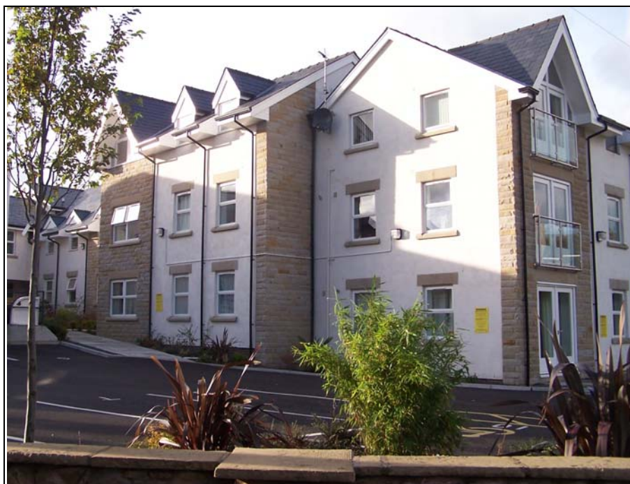
FIGURE 122. NEW REPLACEMENT FLATS
