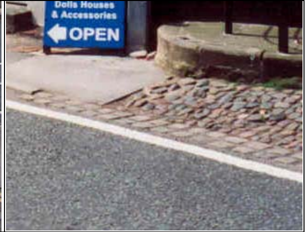
FIGURE 71. A CHANGE IN PAVEMENT MATERIAL FROM CONCRETE TO COBBLES, BRIDGE STREET
