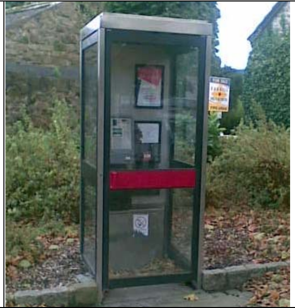
FIGURE 86. MODERN STYLE OF TELEPHONE BOX
