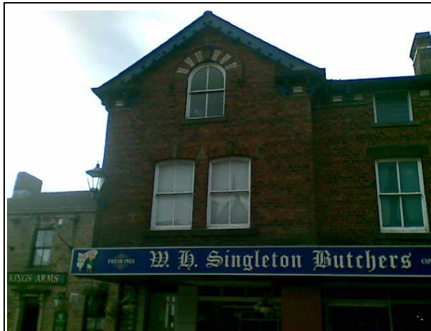
FIGURE 91. RESIDENTIAL UPPER FLOORS OF COMMERCIAL PROPERTY, HIGH STREET
