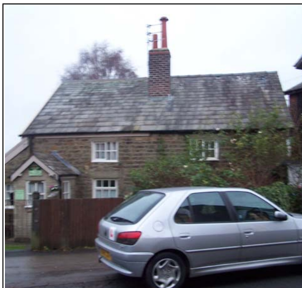
FIGURE 51. SCHOOL COTTAGES, CHURCH STREET
