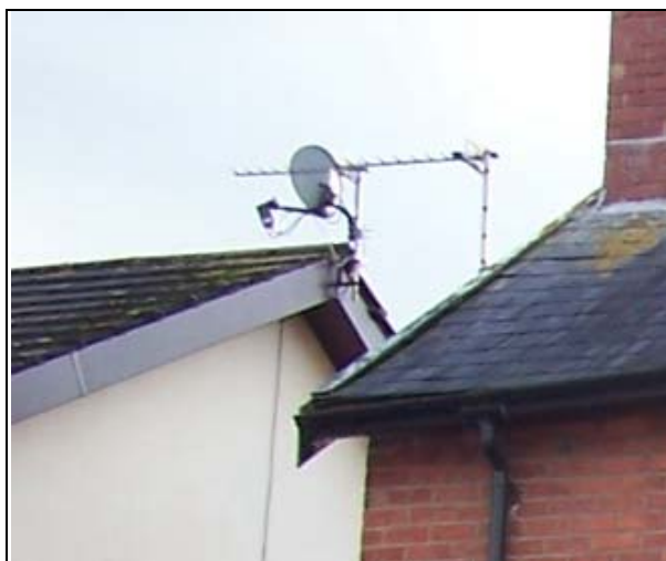
FIGURE 118. INAPPROPRIATELY PLACED SATELLITE DISH
