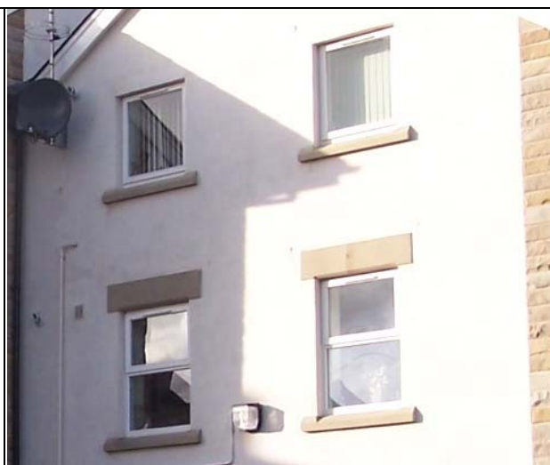
FIGURE 103. MODERN UPVC WINDOWS
