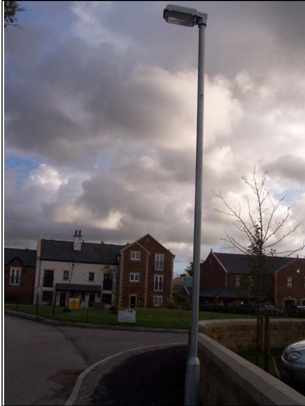
FIGURE 64. INAPPROPRIATE MODERN STREETLIGHT
