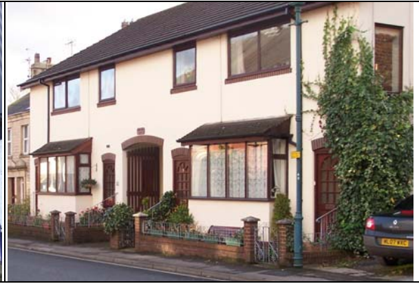
FIGURE 94. RESIDENTIAL BUILDING ON BRIDGE STREET
