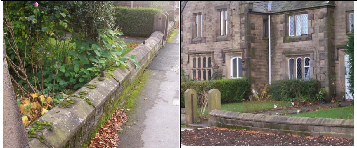
FIGURE 60. BOUNDARY WALLS ON CHURCH STREET FIGURE 61. BOUNDARY WALLS
