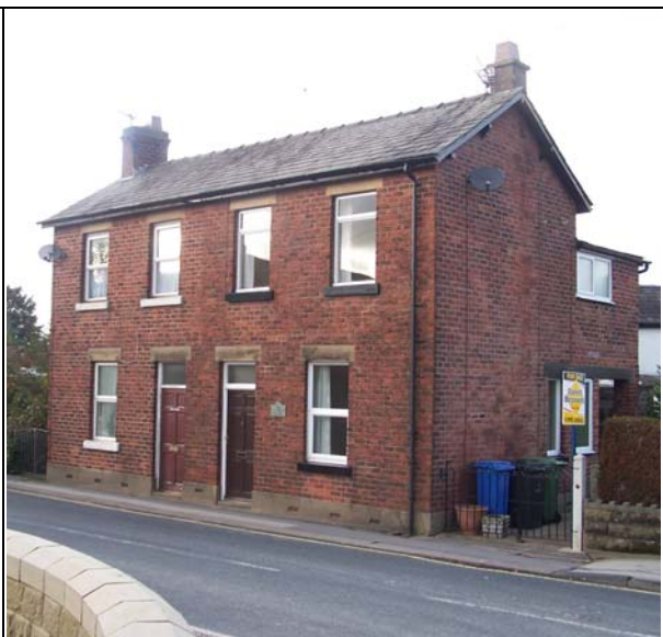
FIGURE 50. MYRTLE COTTAGES, CHURCH STREET
