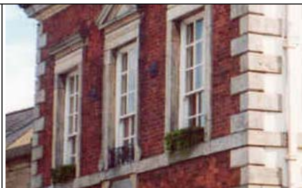
FIGURE 111. GOOD EXAMPLE OF A SASH AND CASEMENT WINDOWS
