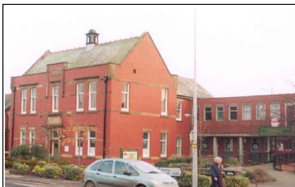
FIGURE 47. COUNCIL OFFICES, VICTORIA TERRACE
