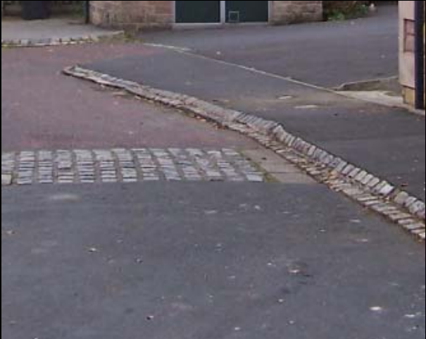
FIGURE 43. SETTS WITHIN MODERN DEVELOPMENT
