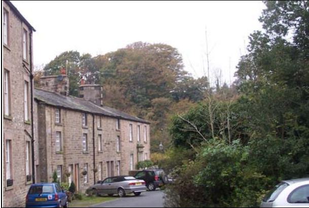
FIGURE 21. VIEWS TOWARDS THE BRIDGE FROM THE SOUTH
