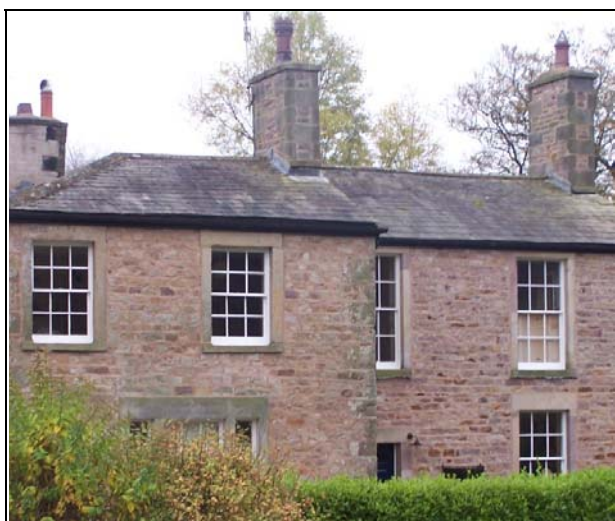
FIGURE 53. SASH AND CASEMENT WINDOWS STILL IN SITU
