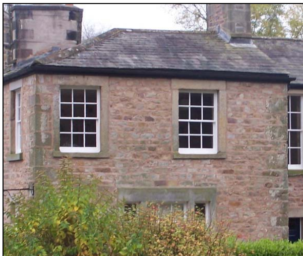
FIGURE 55. TIMBER SASH AND CASEMENT WINDOWS IN SITU
