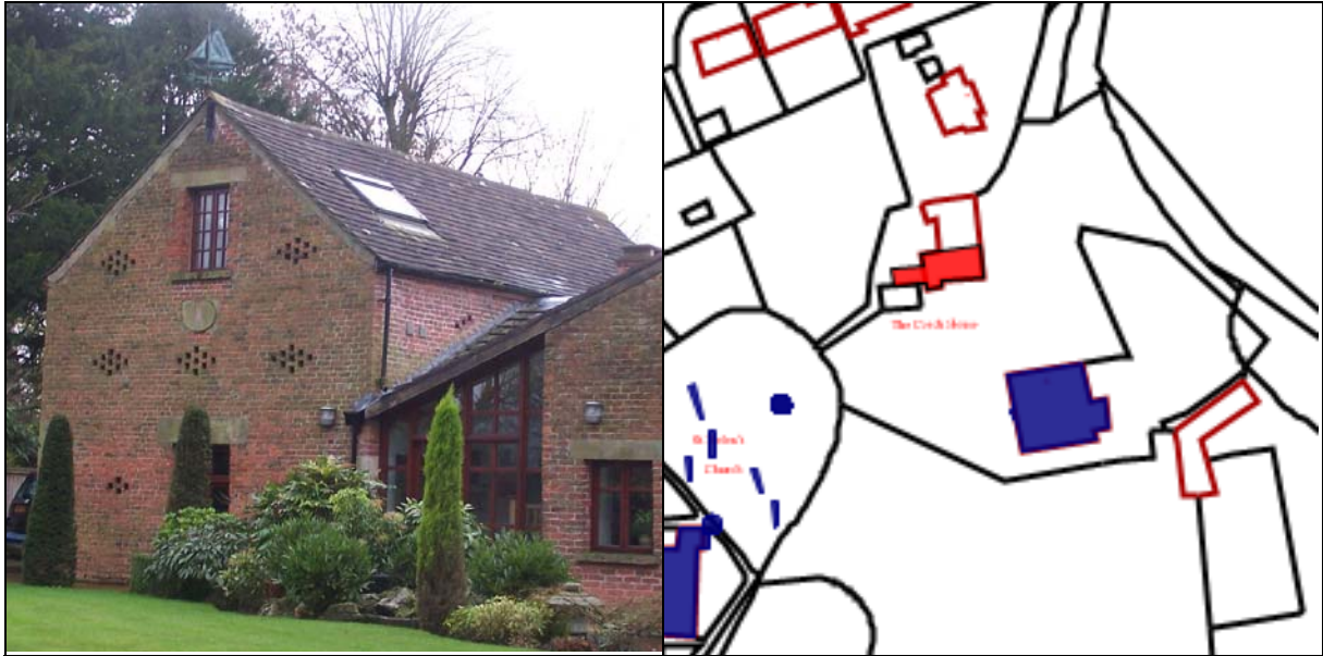
FIGURE 15. BARN NORTH WEST OF OLD VICARAGE
