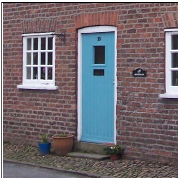
FIGURE 91. TRADITIONAL TIMBER DOORWAY
