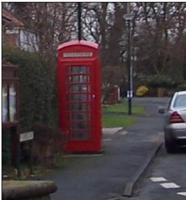
FIGURE 80. K6 STYLE OF TELEPHONE BOX
