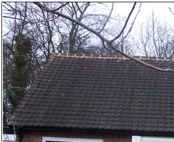
FIGURE 87. MODERN CONCRETE TILE ROOF
