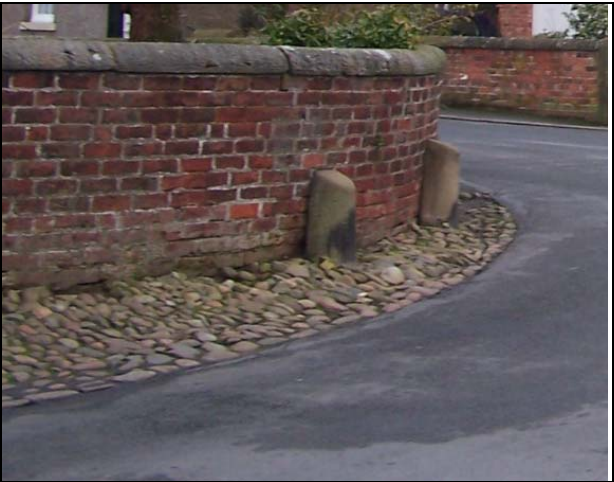
FIGURE 70. ROAD SURFACING BORDERED BY ROUNDED COBBLES
