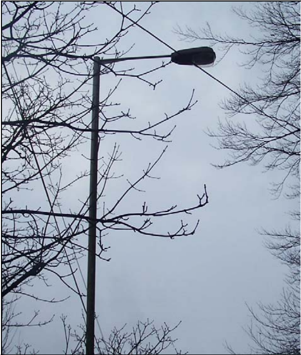
FIGURE 67. MODERN STYLE OF STREET LIGHTING
