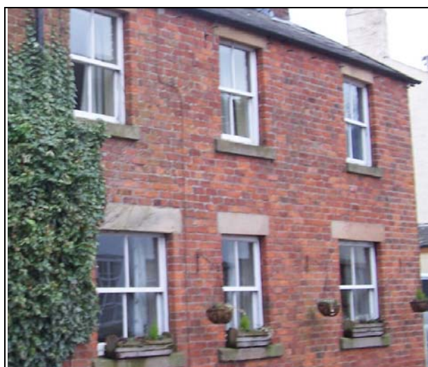
FIGURE 97. APPROPRIATE SASH AND CASEMENT WINDOWS
