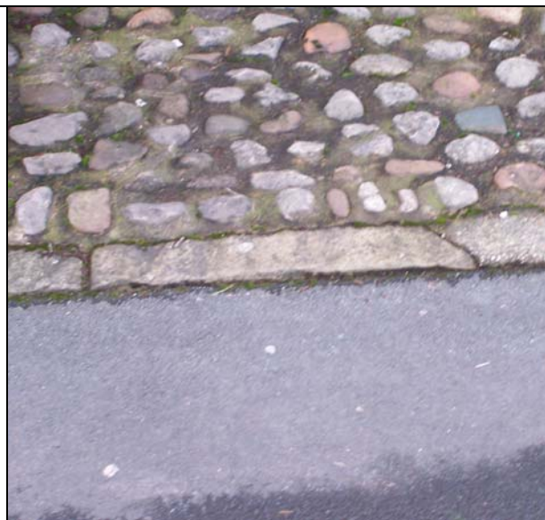
FIGURE 72. VARIATION IN PAVEMENT MATERIALS
