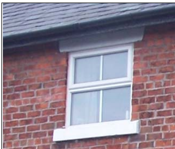
FIGURE 93. MODERN UPVC WINDOWS
