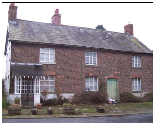
FIGURE 47. MANOR HOUSE AND MANOR COTTAGE
