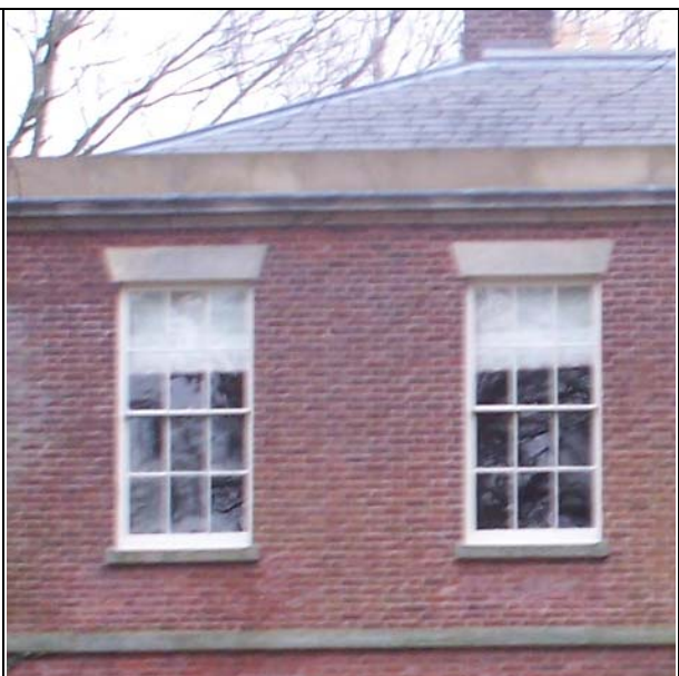
FIGURE 90. TIMBER SASH AND CASEMENT WINDOWS
