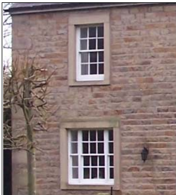
FIGURE 95. GOOD EXAMPLE OF SASH AND CASEMENT WINDOWS
