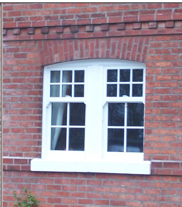
FIGURE 96. GOOD EXAMPLE OF A SASH AND CASEMENT WINDOWS
