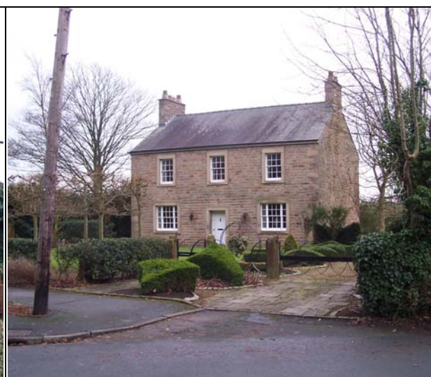
FIGURE 84. TRADITIONAL NATURAL STONE BUILDING
