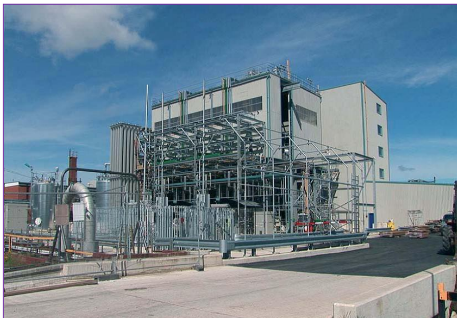
Hillhouse Technology Enterprise Zone, Thornton
