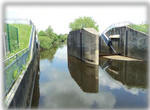
Flood Barrier on Wyre near Millennium Green
