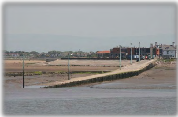
Knott End Ferry Slipway
