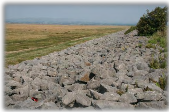
Rock riprap adjacent to slipway
