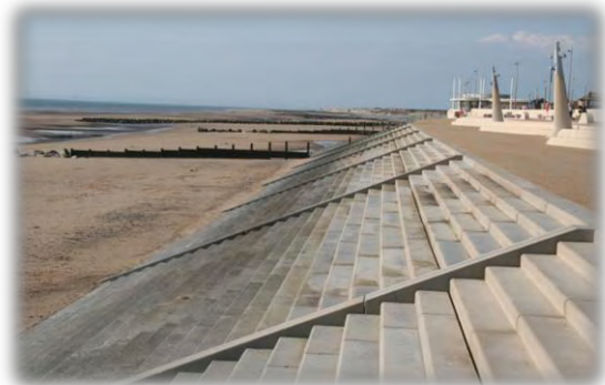
Promenade revetment steps with good access
