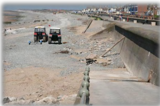
Ongoing Beach maintenance
