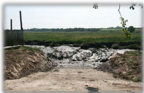
Newly constructed slipway
