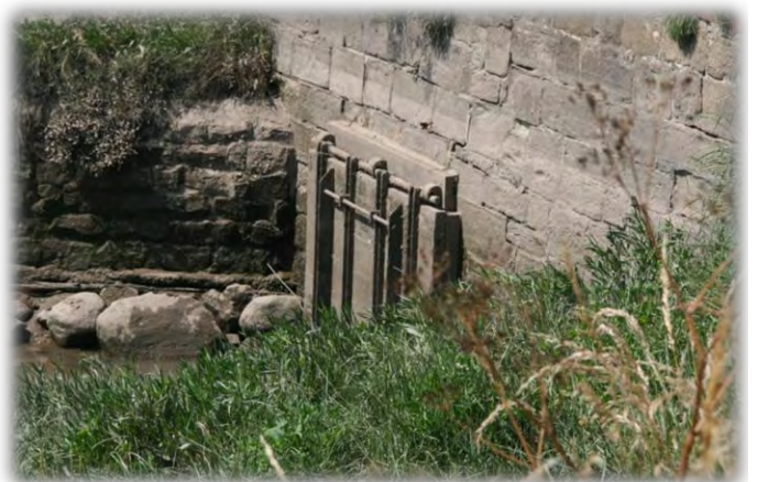
The Tidal Barrier beneath the road bridge
