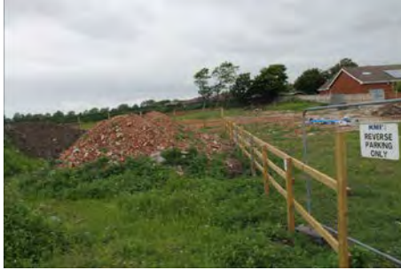
Photo 22.2 (looking north west)
