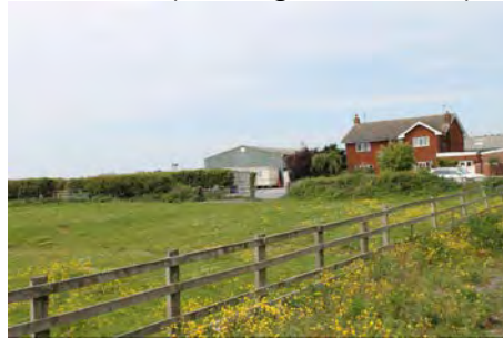
Photo 5.2 (looking north west)
