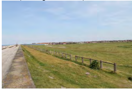
P1.2 (looking north east)
