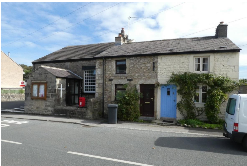
Hollins Lane Methodist Church and two adjoining terraced cottages on Hollins Lane (approx. 280 m north of site)
