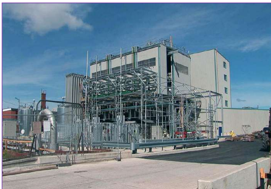
Hillhouse Technology Enterprise Zone, Thornton
