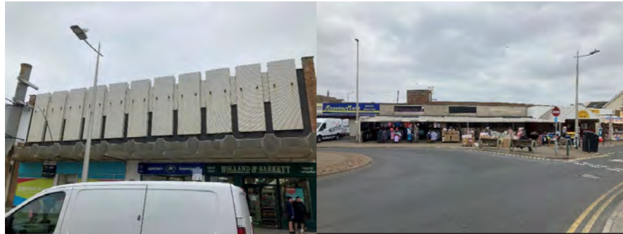
Site photo show poor quality retail frontage along Victoria Road West
