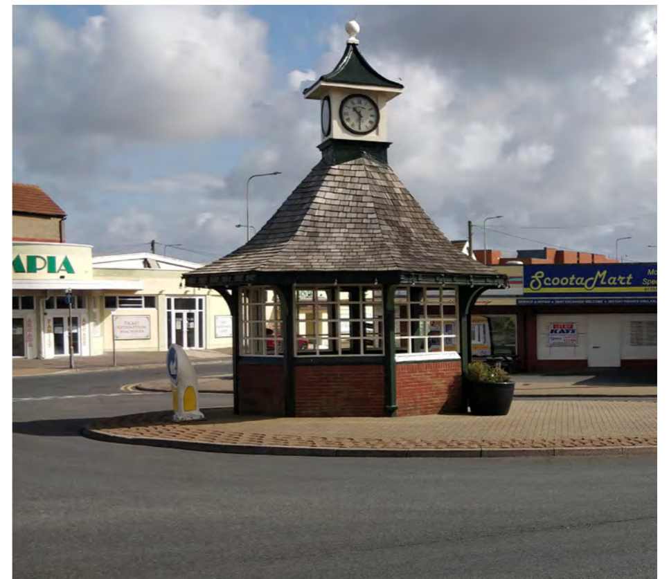
Site photo of the Roundabout Shelter at the end of Victoria Road West
