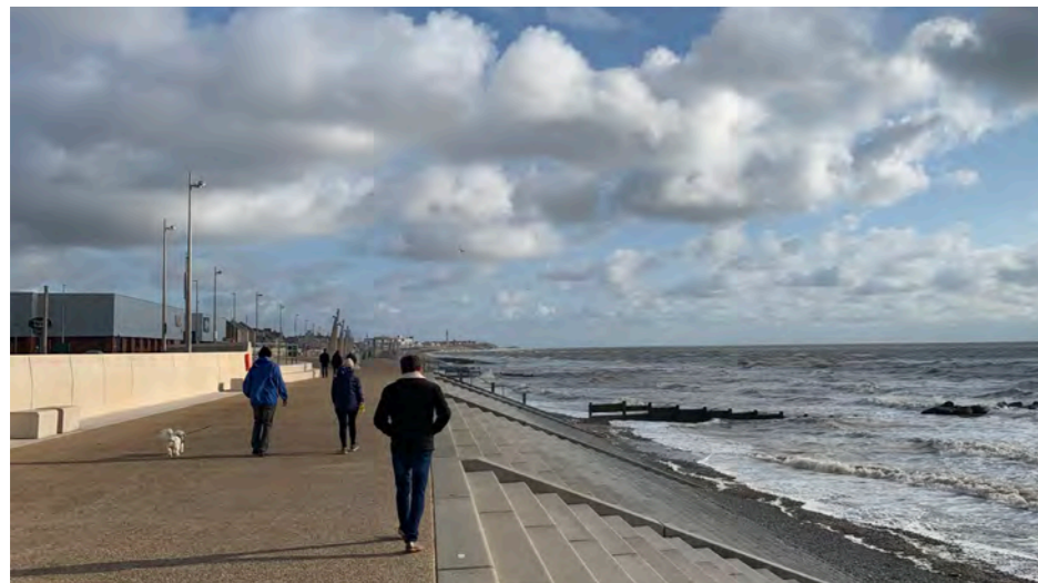
Site photo showing a view from the promenade facing south
