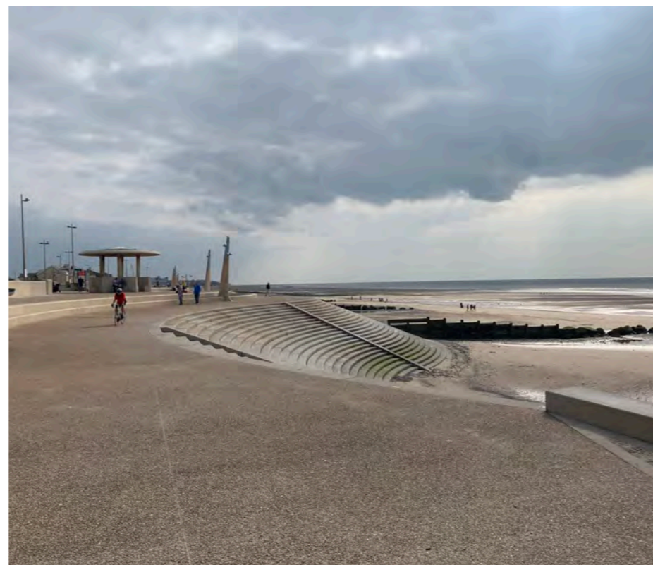
Site photo of the top of Cleveleys Promenade looking to the south
