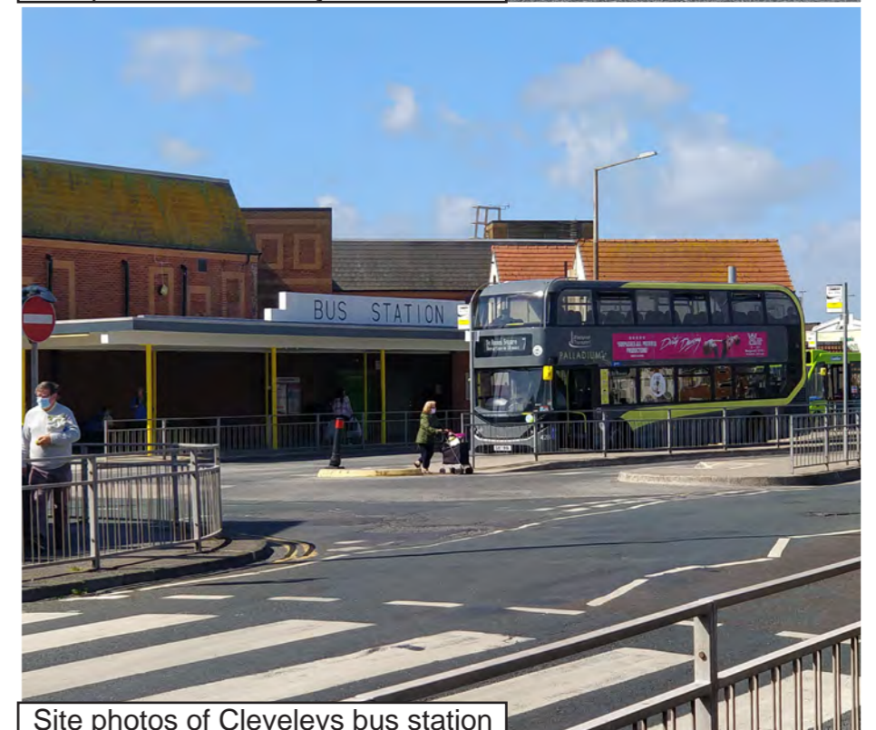
Site photos of Cleveleys bus station
