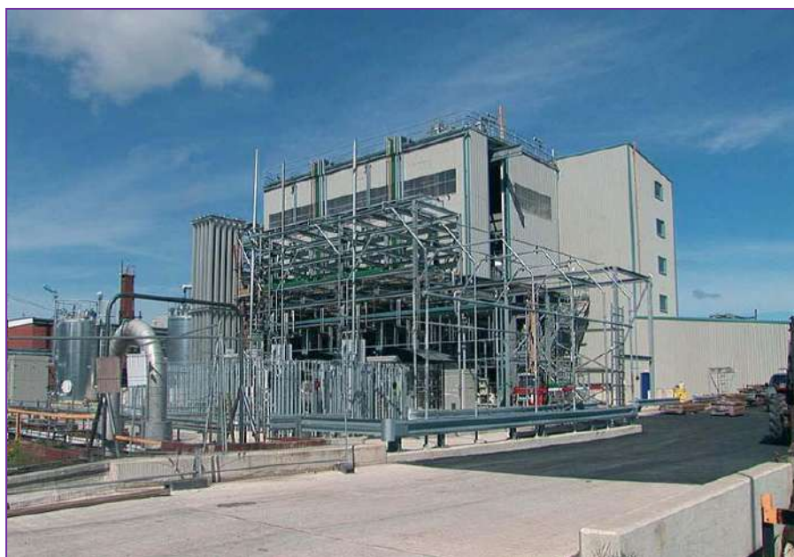
Hillhouse Technology Enterprise Zone, Thornton
