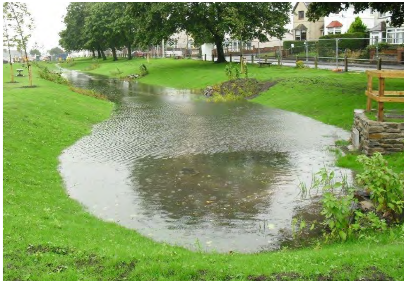
Example of swale
