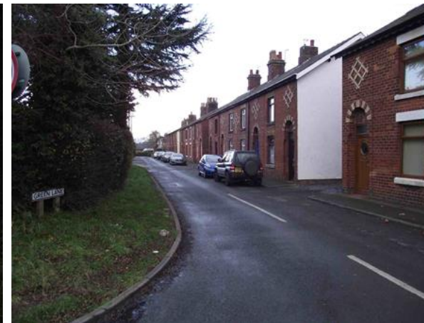
7. Terraced housing to Green Lane
